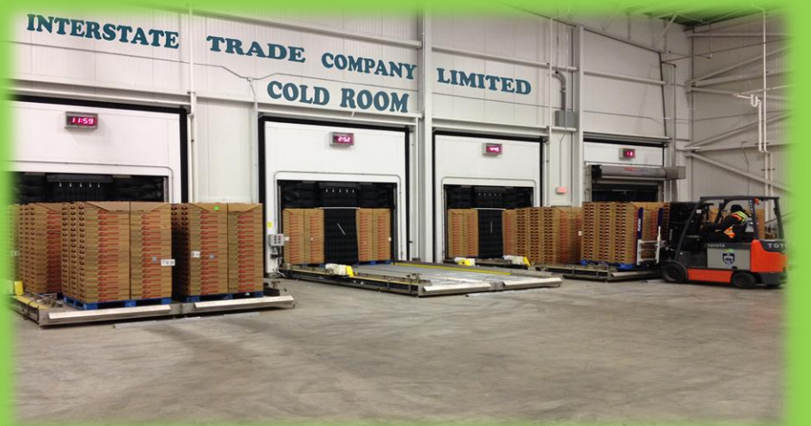
ITC storage cold room
